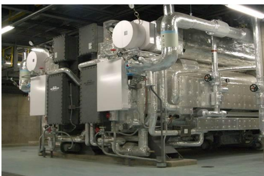
蒸気吸収冷凍機(AR-2A・AR-2B)
