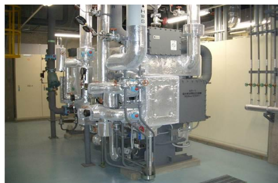
温水吸収冷凍機(AR-1)
